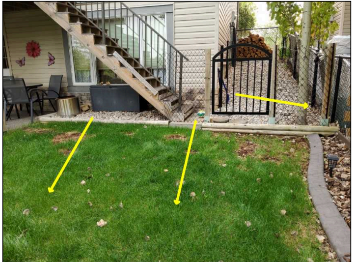
Regrading where needed is recommended to assure all water drains away from the home foundation at all times.
