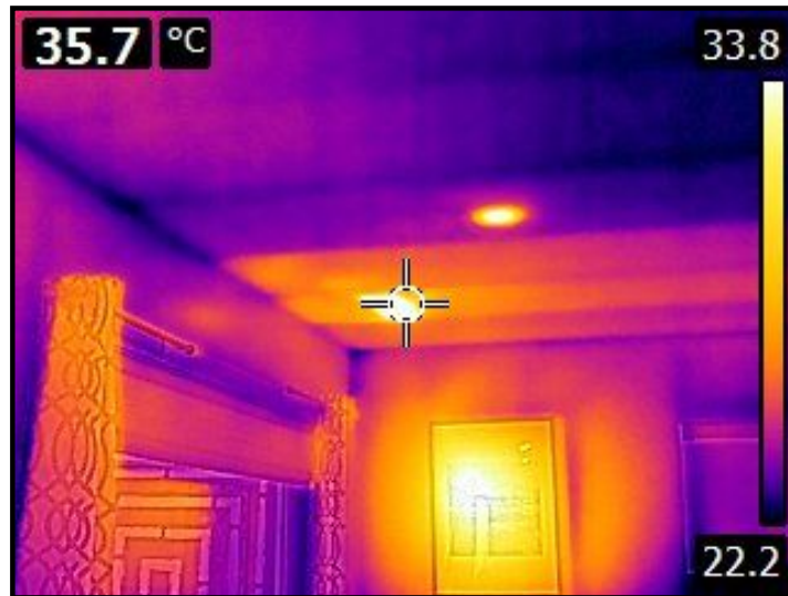
Basement heating register, responding to test
