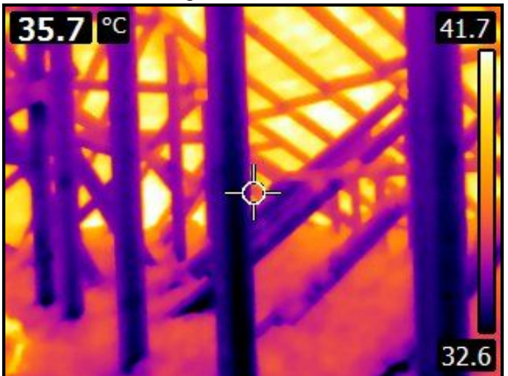
Visibly inspected in attic area from ladders edge on thermal scan
