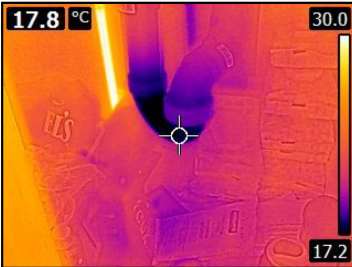
Limited thermal scan due to storage of personal property.
