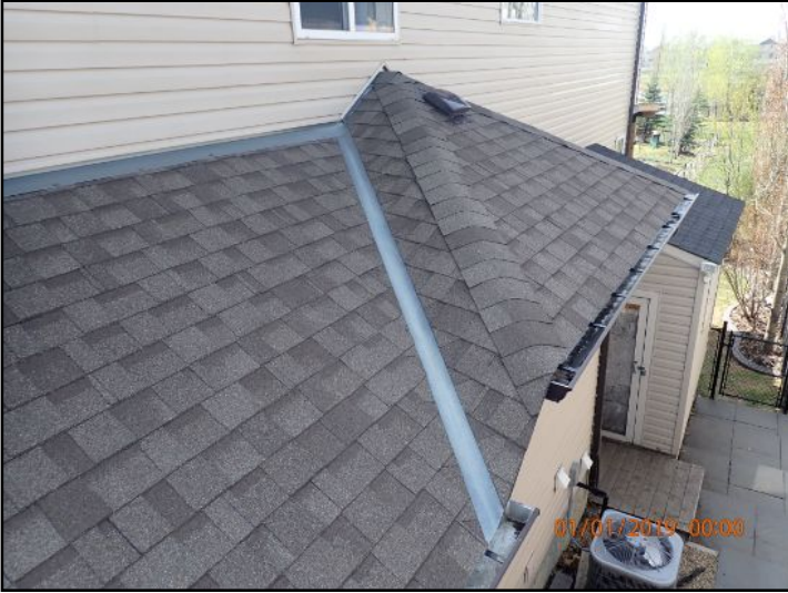
Lower Front Roof
