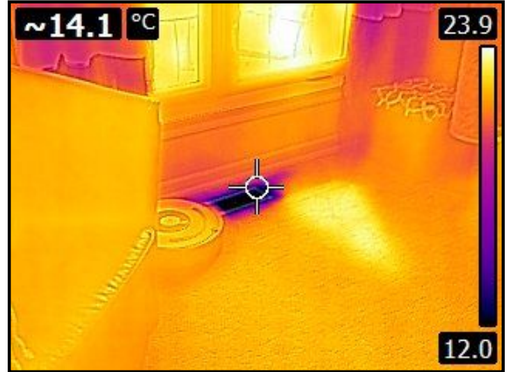
Main Level A/C responding to test at the time of the inspection
