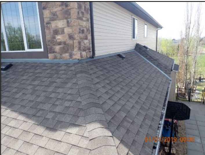
Lower Front Roof
