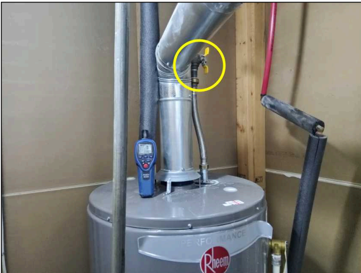
Water shut off circled.
