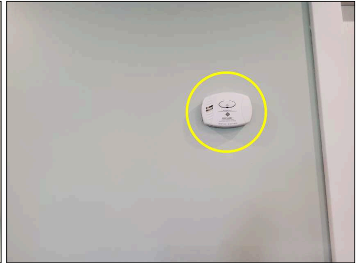
Carbon monoxide detectors in place and worked on testing, (CO detectors only have a 7 year life span, if age unknown suggest replacing)
