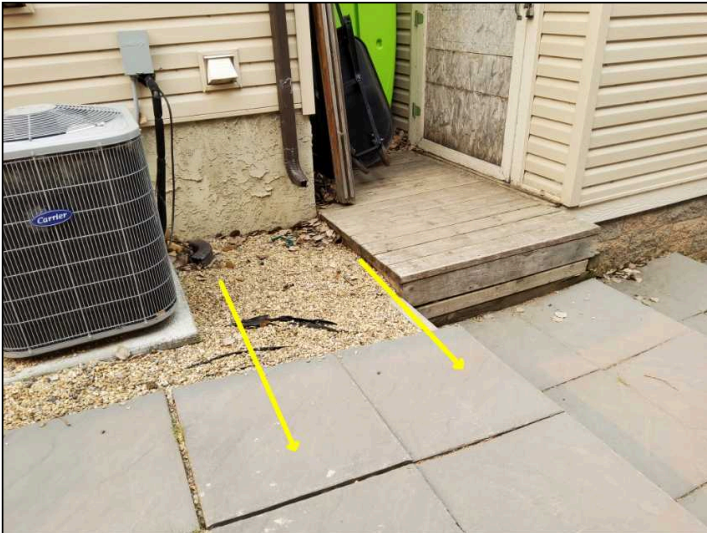
Regrading where needed is recommended to assure all water drains away from the home foundation at all times.
