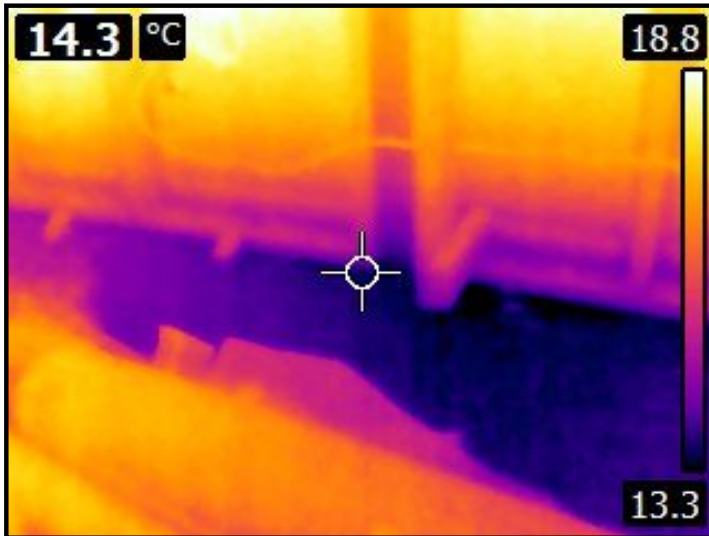
Under stair storage area
