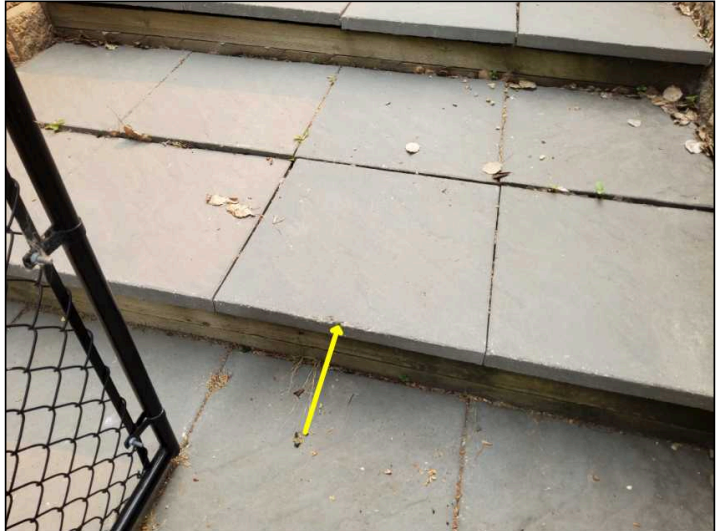
Loose paver tiles observed, possible trip or fall hazard, recommend review for repair
