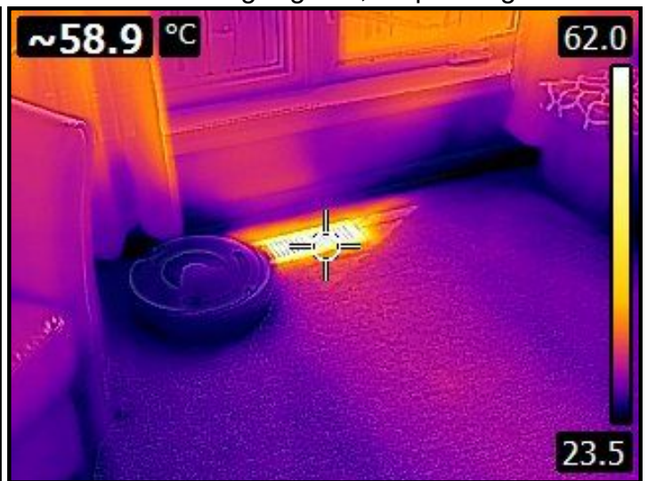
Various heat registers are tested with thermal imaging for consistency.
