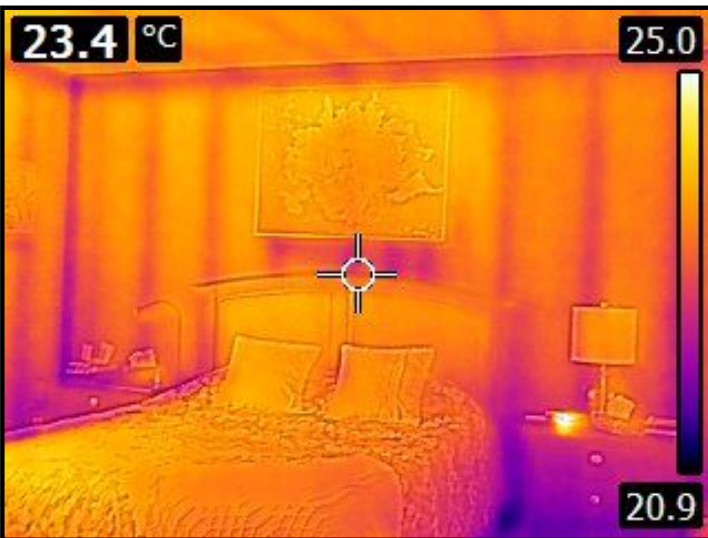
Primary Bedroom - Thermal Image
