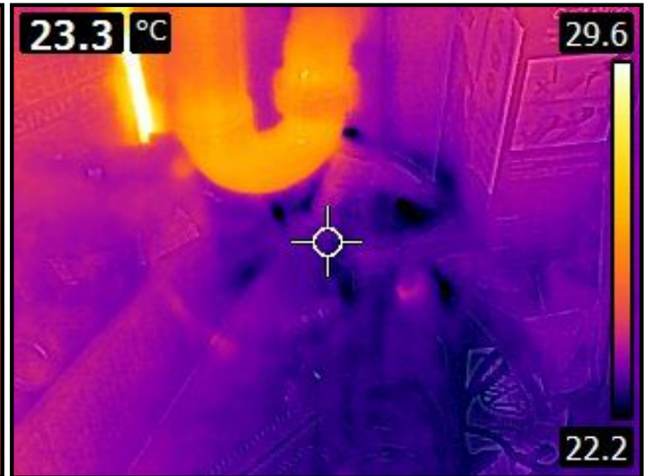
No leaks observed during the inspection.
