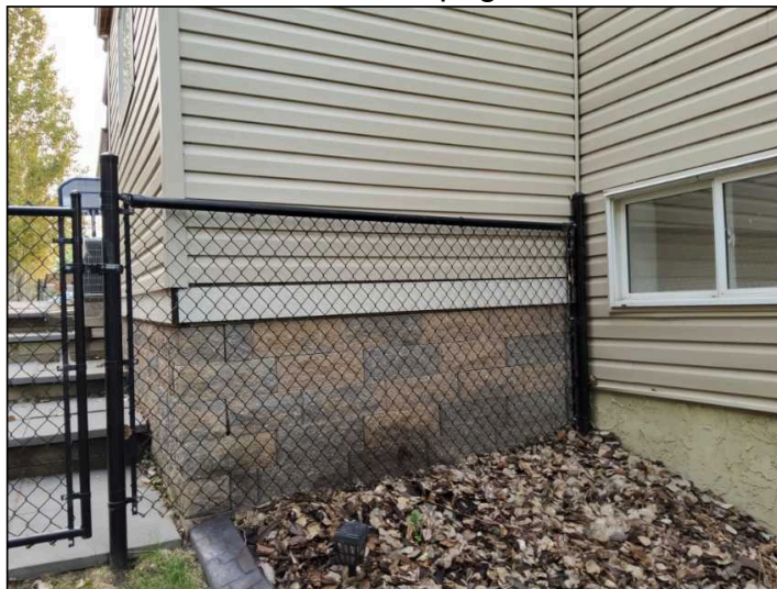
Limited inspection due to personal property, sheds and vegetation.
