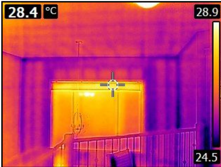
Upper landing thermal image
