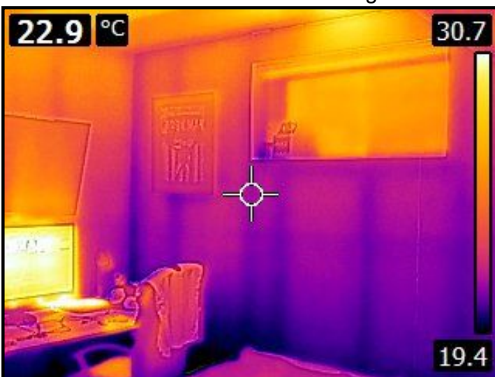
Basement Bedroom - Thermal Image
