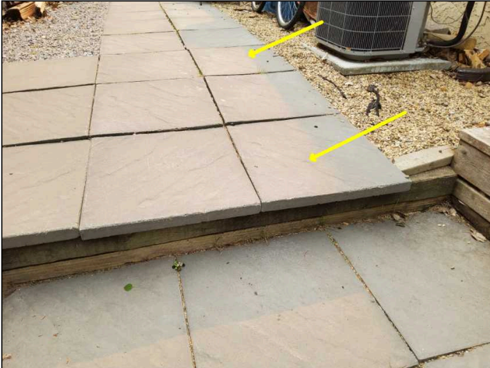
Loose paver tiles observed recommend review for repair
