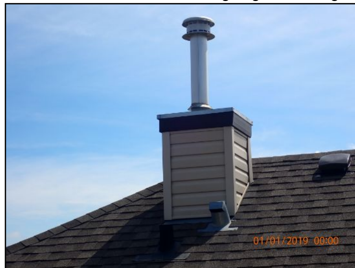
Peeling paint observed, recommend resealing to prevent moisture intrusion
