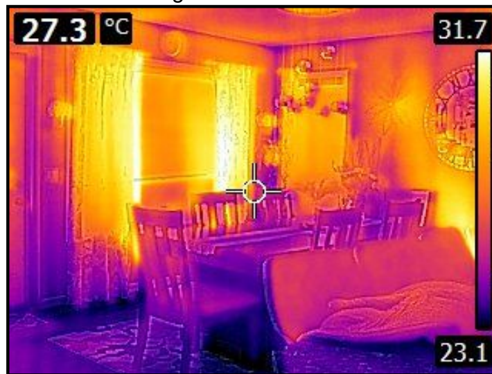
Dining Area - Thermal Image
