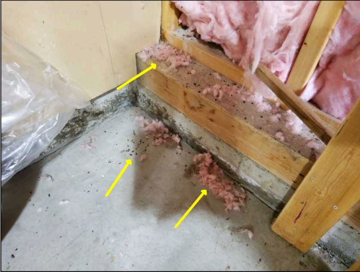
Indication of possible pest activity observed, recommend further review by a certified pest control if concerned
