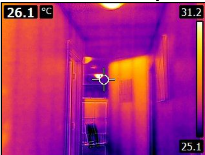
Upper landing thermal image
