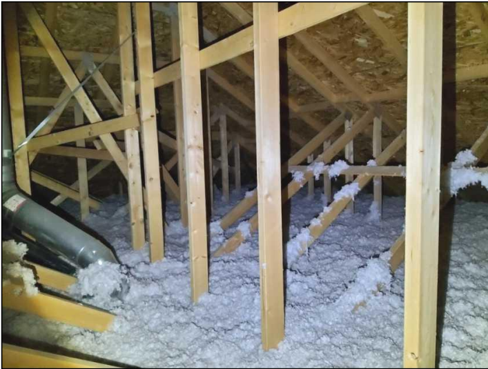
Visibly inspected in attic area from ladders edge with flash light
