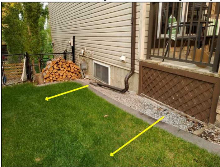
For correct drainage around the home all sides would slope away from the home, this assists in preventing water from sitting at the foundation wall.
