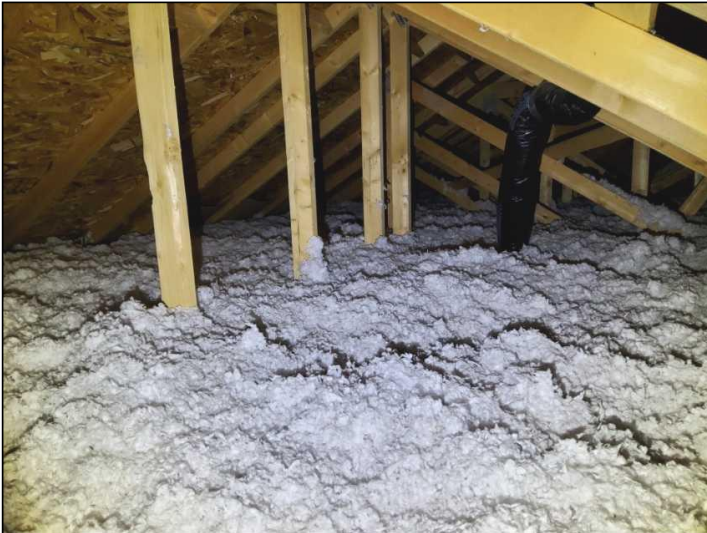
Limited review due to insulation installed between the rafters.
