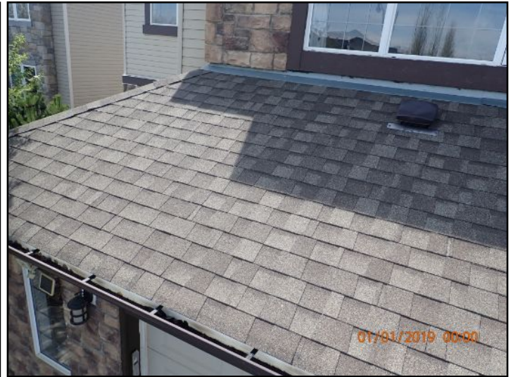
Lower Front and Garage Roof
